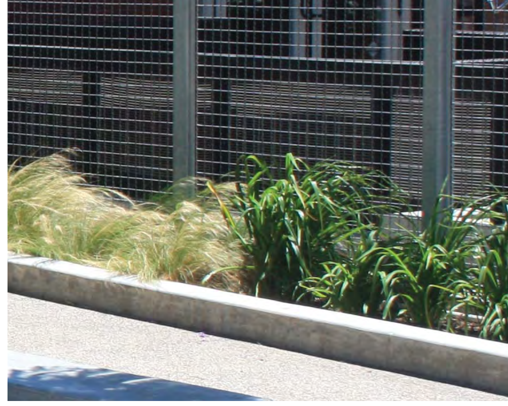
Concrete Planter Curb
